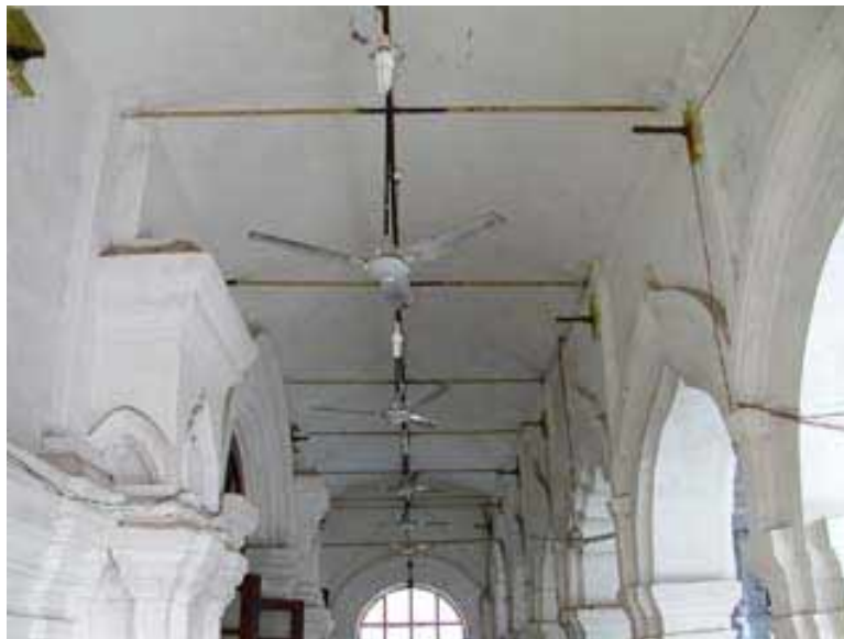
Figure 5. Retrofitting of an old Mosque using tie rods at Aberdeen, Port Blair.
