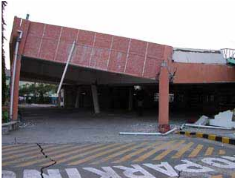
Figure 1. Partially collapsed Passenger Terminal Building at Haddo Wharf, Port Blair.
