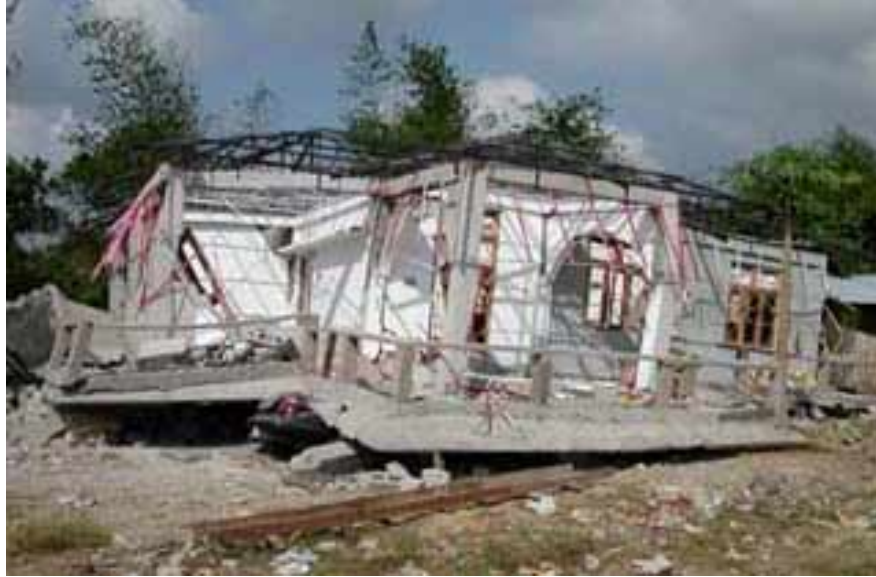
Figure 4. Collapsed 2-storey RC building on stilts at Bamboo Flat near Port Blair.
